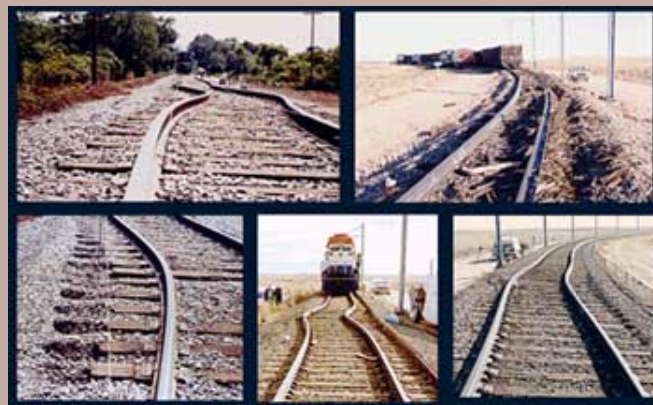
Figure 9.8: Train track buckling. (US Department of Transportation)
